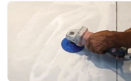
STEP 1 : GRINDING
