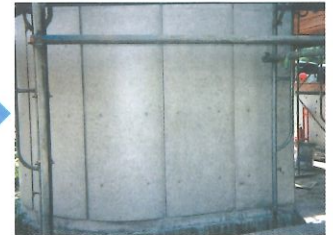
After Application of Waterbase AC system
