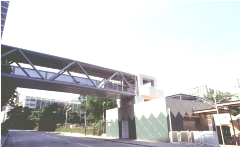
▲ Footbridge at Sheung Shing St., Homantin
